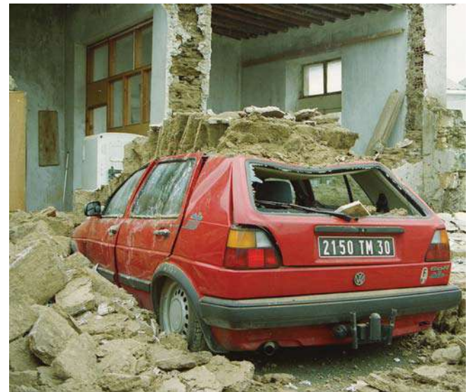
PSA RIBBON COLLAPSED 3 Steven Stavri Cyprus
