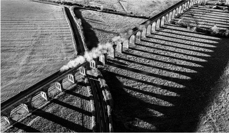
GPU Ribbon Harringworth Viaduct Roger Newark United Kingdom
