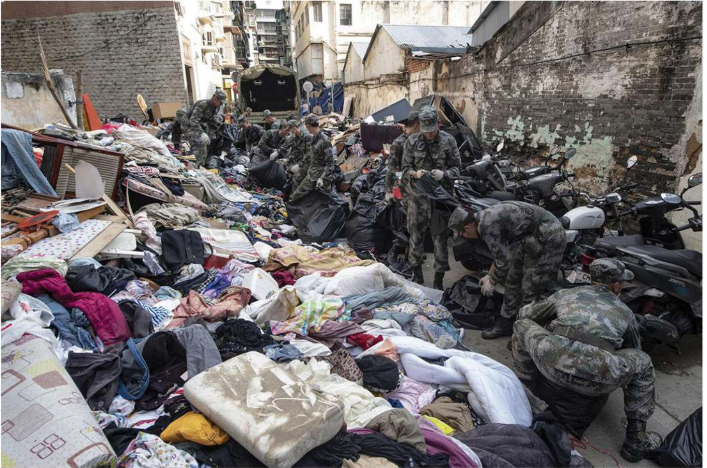
GPU Bronze Post Disaster Clean up Tak Cheong Pun Macau, China
